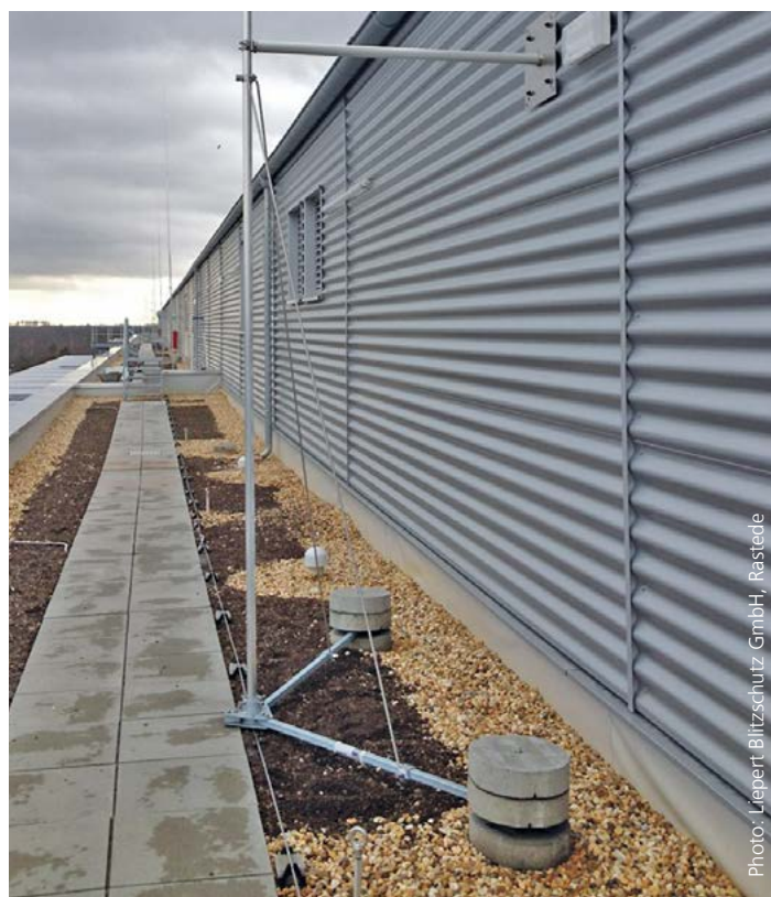
Tripod for use as wall-mounted two-legged stand
