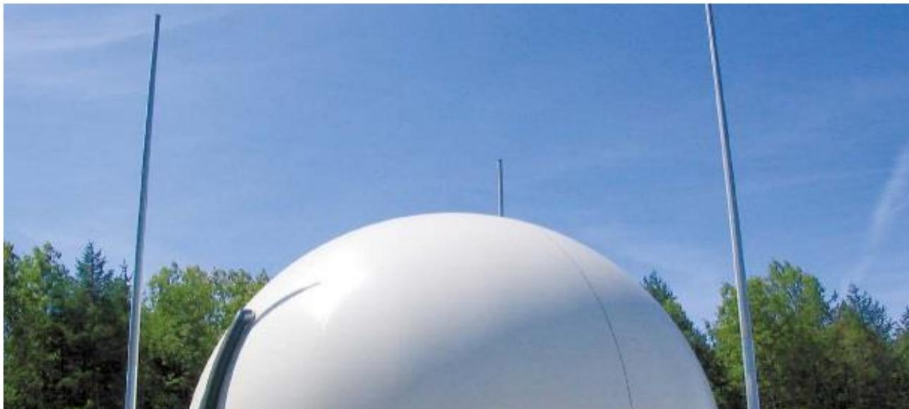
The risk of a lightning strike can only be mitigated against if a lightning protection system is fitted following from a risk assessment to BS EN 62305 being carried out. Both BS EN 62305-2 and BS EN 1127 gives a starting point of a level 2 lightning protection system. This will recommend or strongly encourage the deployment of an isolated lightning protection system, not a cross bonded system.
