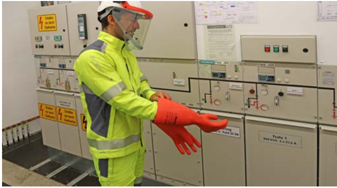
Work on live parts with insulating gloves.
