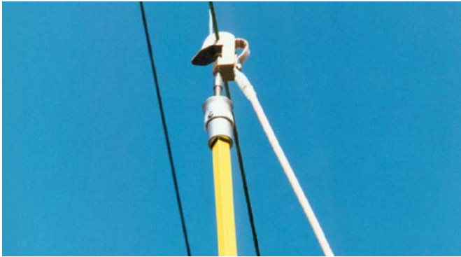
Coupling the earth clamp to the overhead contact line.
