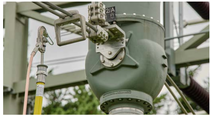
Attaching a phase screw clamp to an overhead line.
