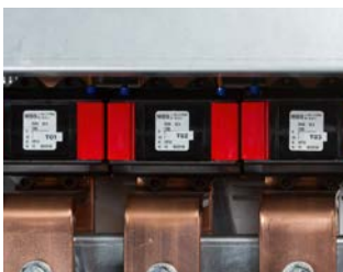
Built-in protective current transformers
