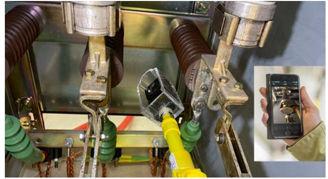
System monitoring with wireless inspection camera and live display on a smartphone.
