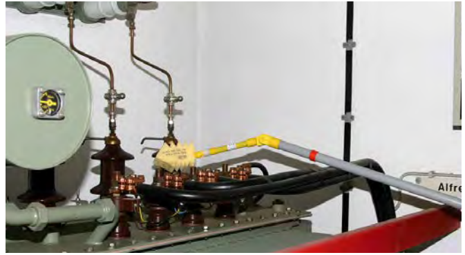
Damp cleaning of a transformer using the FRS ZK MS damp cleaning kit.
