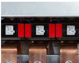
Built-in protective current transformers
