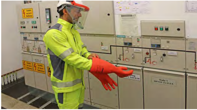
Work on live parts with insulating gloves.
