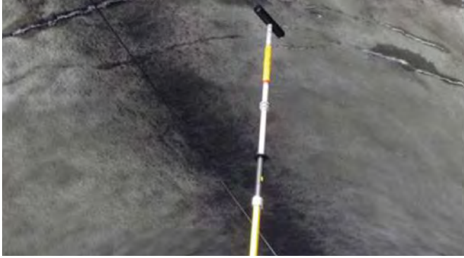
Removing icicles on a tunnel entrance.
