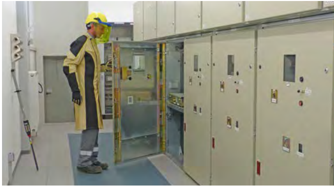
Switch room with insulating mat fitted.
