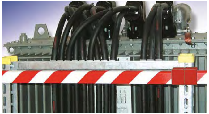
Barrier in a transformer station.
