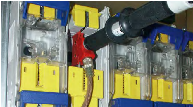
Attaching a fully insulated earthing and short-circuiting device using an earthing handle of type VI.
