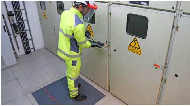
Switch room with insulating mat fitted.
