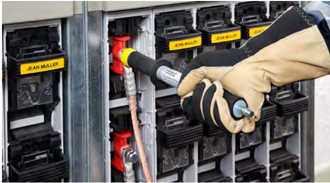
Attaching a partly insulated earthing and short-circuiting device using an earthing handle of type TI.
